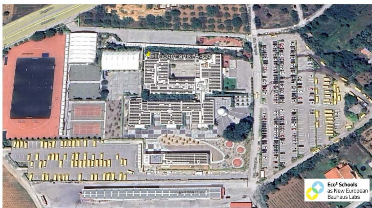
Figure 1. EA School – Main campus after the completion of certain renovation works. Solar panels that will contribute to the energy efficiency of the school are visible on the roof of the building.
