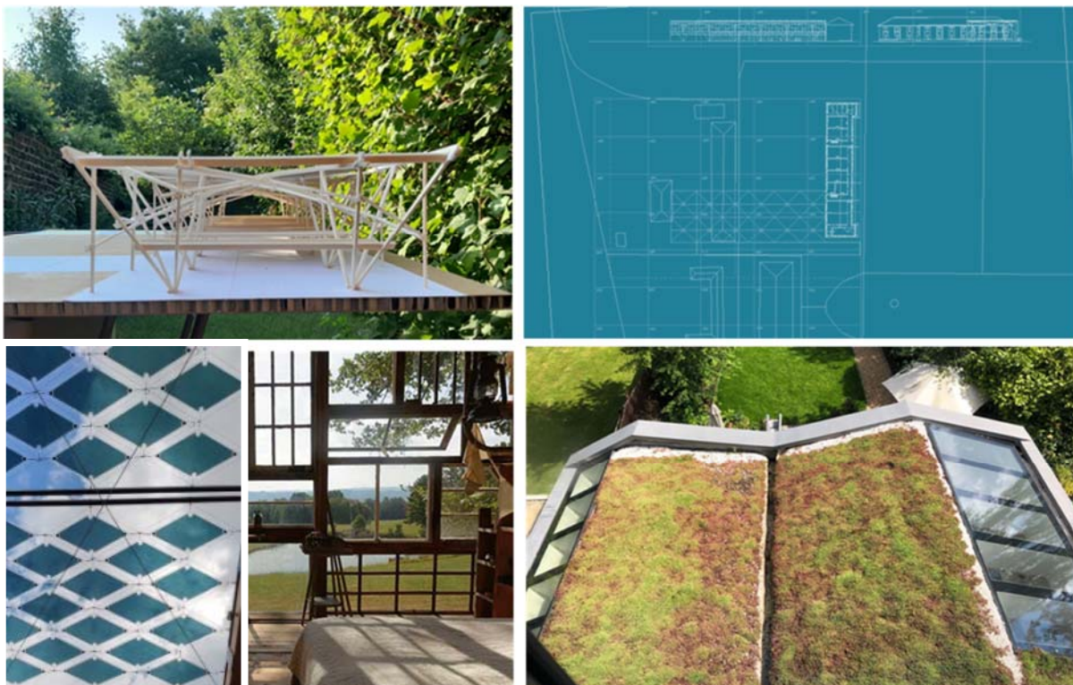
Figure 6. Illustration: scalable “worksite-school” test activities on Microville112 Pilot Site, a coproduced Bamboo extension that will deliver a multifunctional Green Hall connecting and extending the capacity of the educational third place ECO 2 -Campus M112 (80-90m x26m x11m 2 levels multifunctional greenhouse, local bio sourced net zero bamboo structure, green roof and central rainwater collection, covered by a thin film solar canopy bioinspired textured color to the façades, circular water cistern and basins in the basement, hydroponic indoor plantations and fish farming, glazed facade composed of recycled deconstruction wood frames opening outwards and painted in different colors, new spaces co-learning-action.
