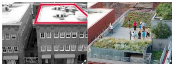
ASLA Headquarters Green Roof, before / after (USA)
